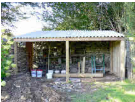
Ross and Josie's new bee house under construction
